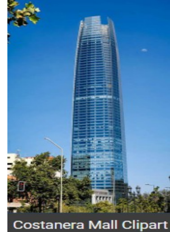
Costanera Center Tower
